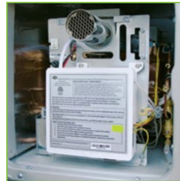
Tankless Water Heater
